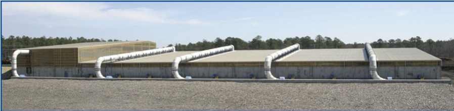
McGill-Waverly is the largest enclosed composting facility in Virginia. In the foreground is the biofilter, designed to remove odors and particulates from process air.
